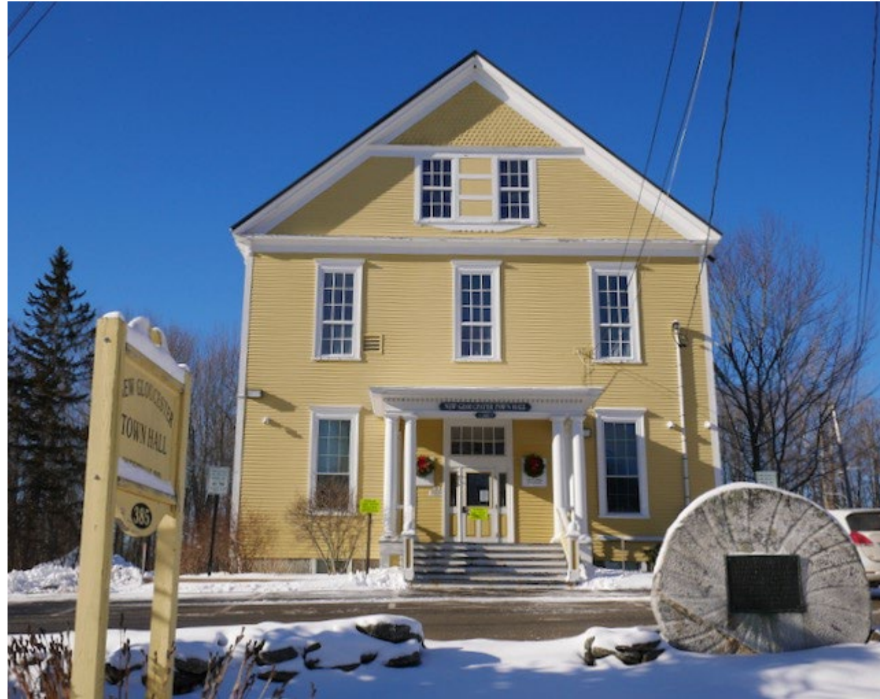
New Gloucester Town Hall
